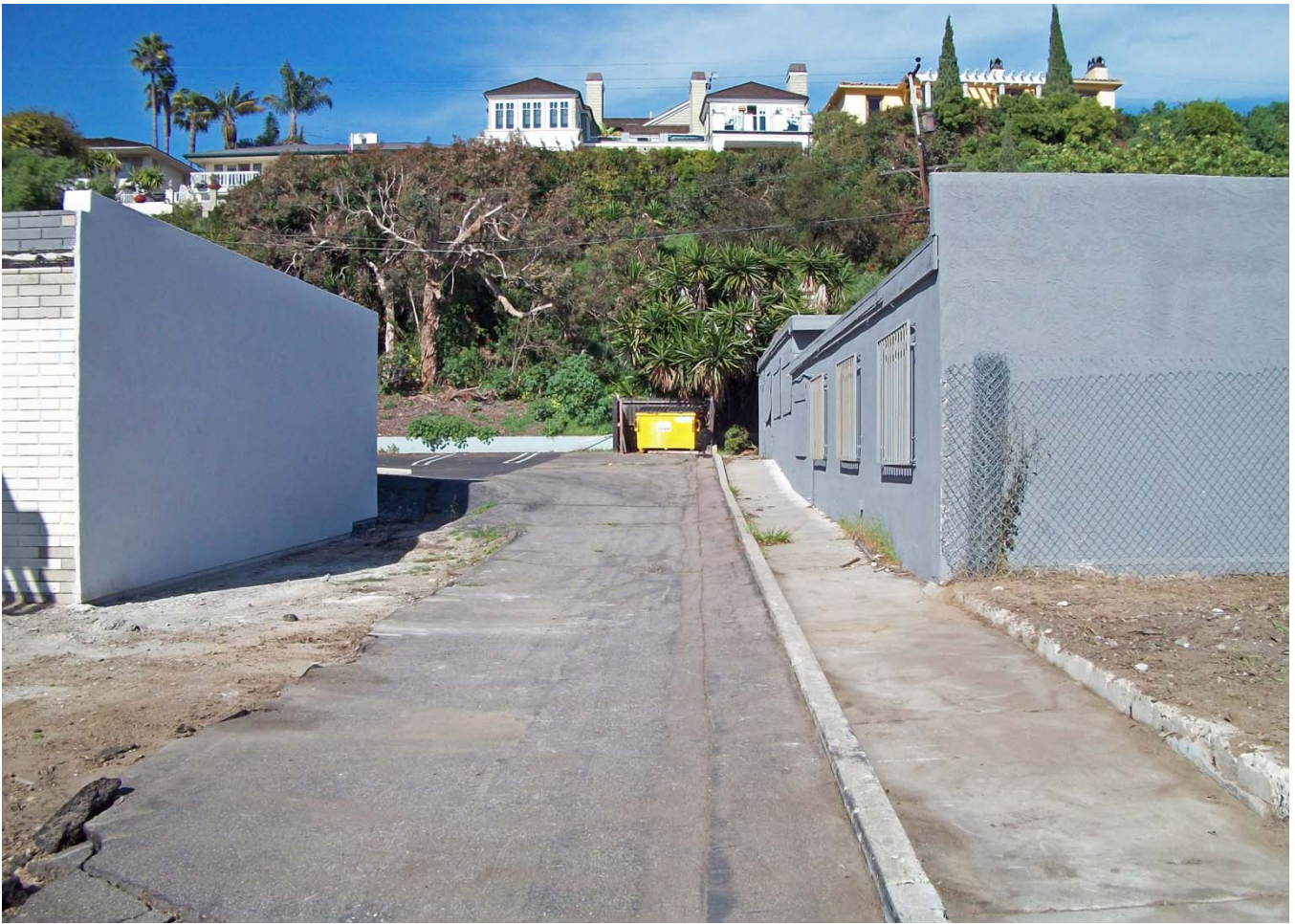
7. Overview of Western Elevation of Project Area from Coast Highway (North).
