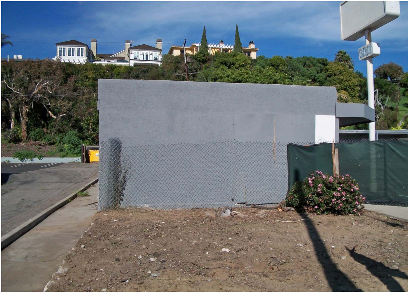
13. View of South Elevation from Southwest Corner (North).
