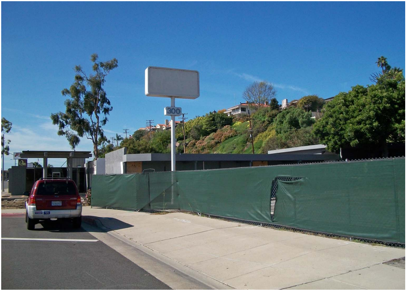
3. Overview of Frontage on Coast Highway (Northwest).
