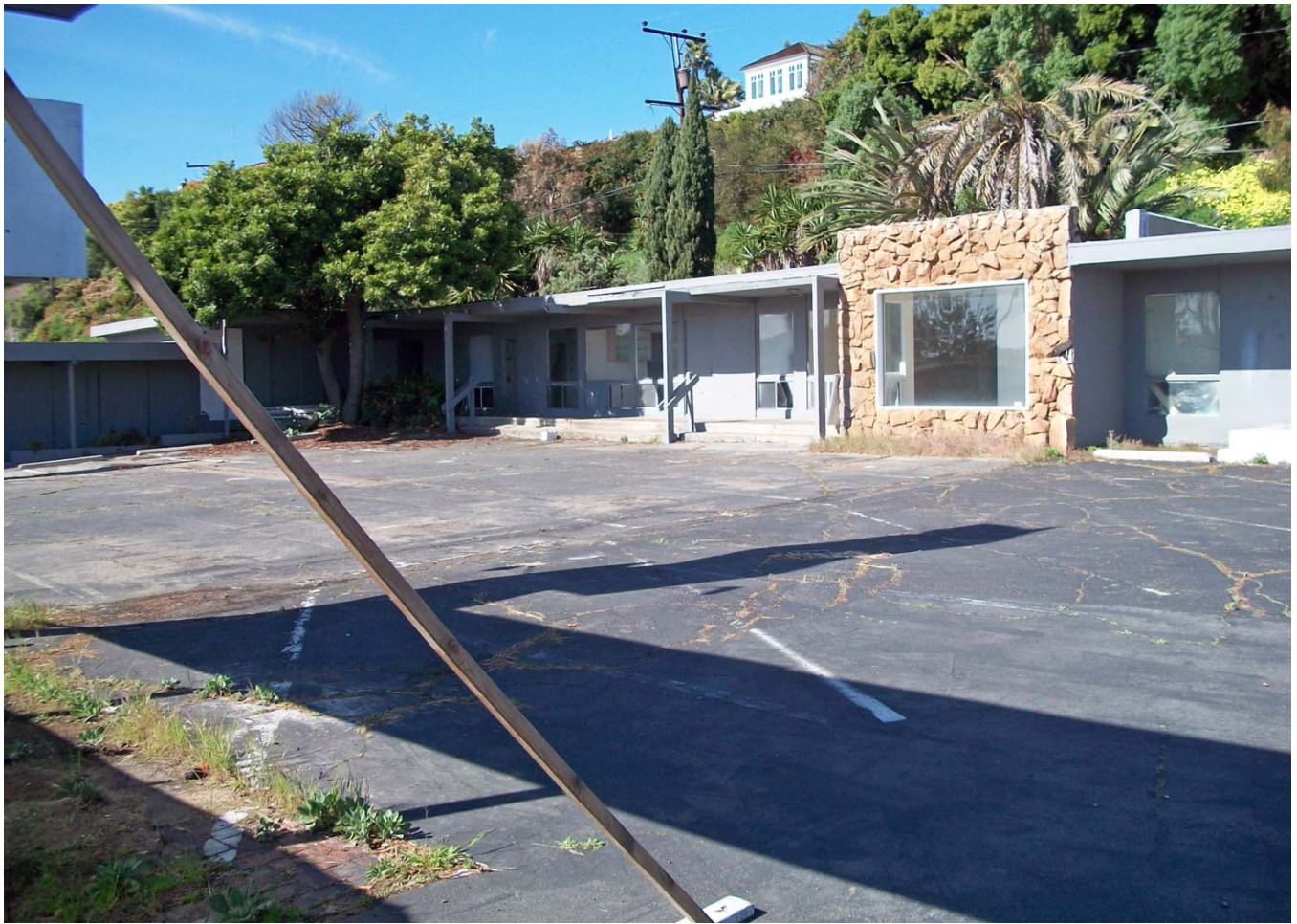
19. Overview of South Elevation from Coast Highway (Northwest).
