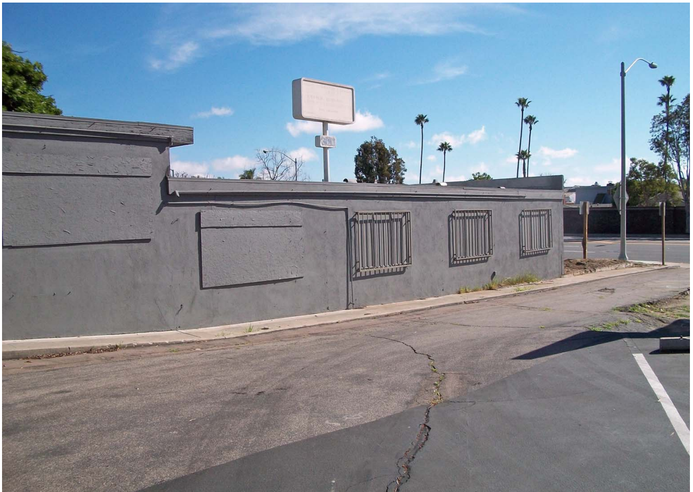
10. Overview of West Elevation from Northwest (Southeast).
