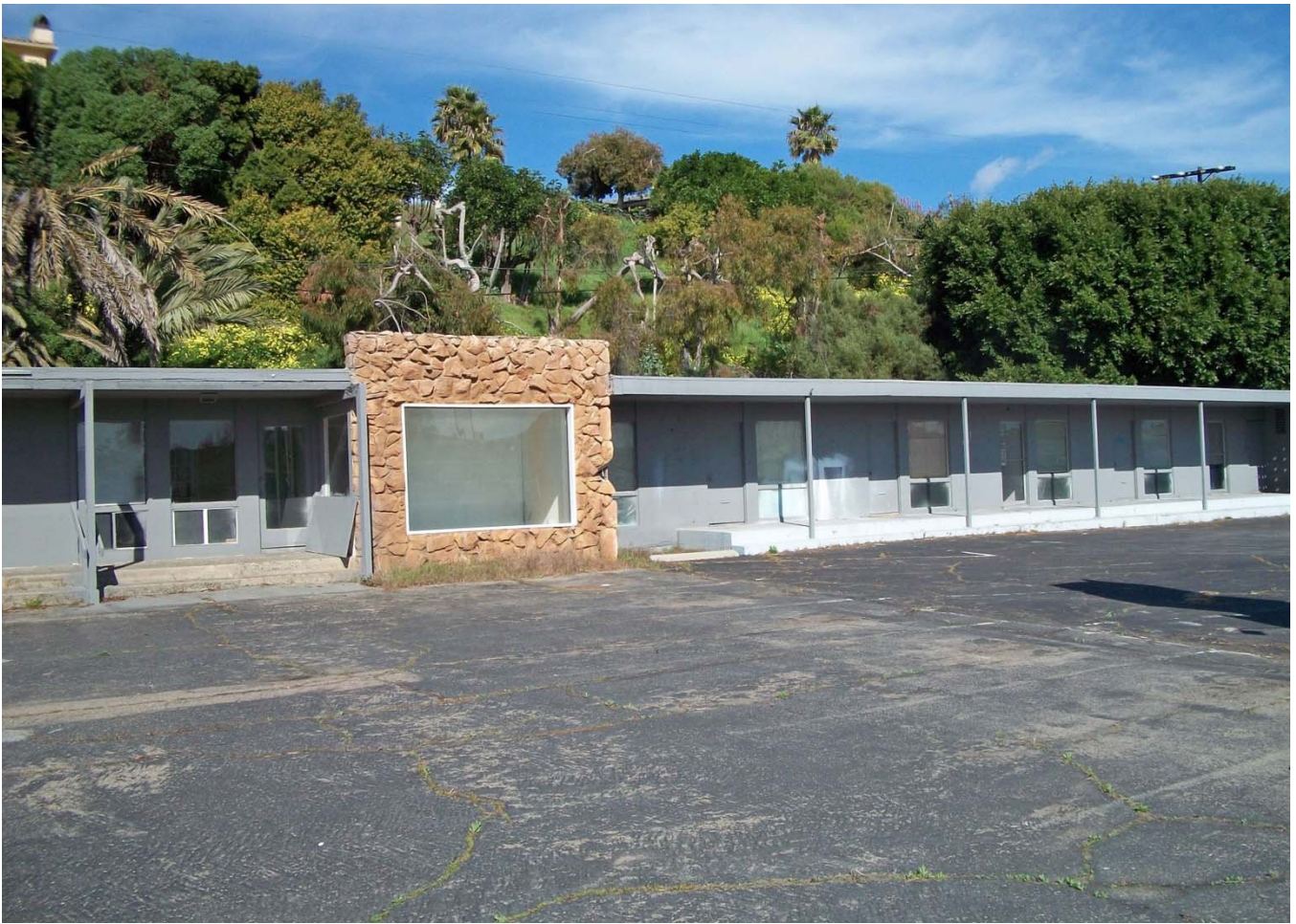
17. Overview of Northern Ell from Coast Highway (North/Northeast).
