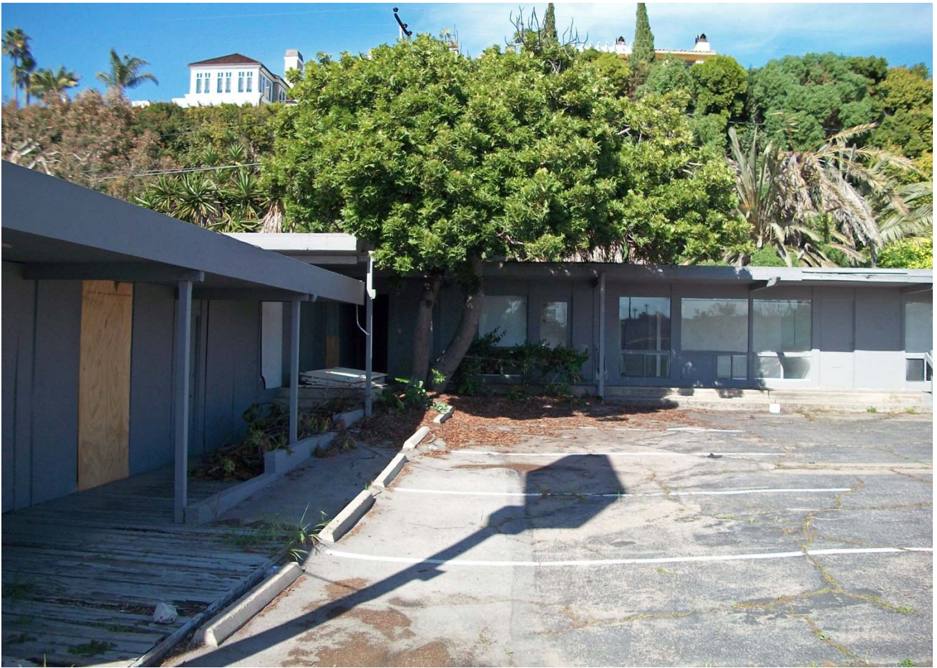
15. Interior Corner of Buildings from Coast Highway (North).
