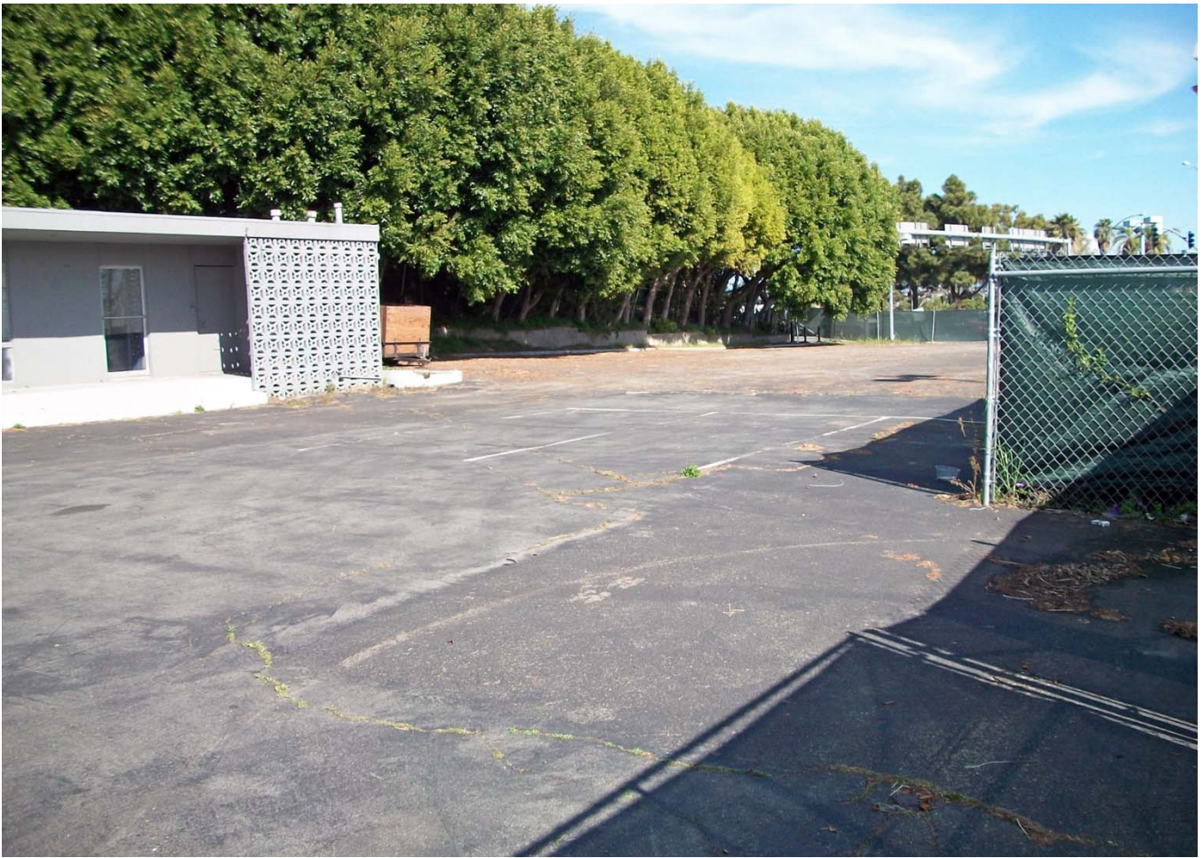
21. Overview of Parking Area Located to East of Building Complex (East/Northeast).
