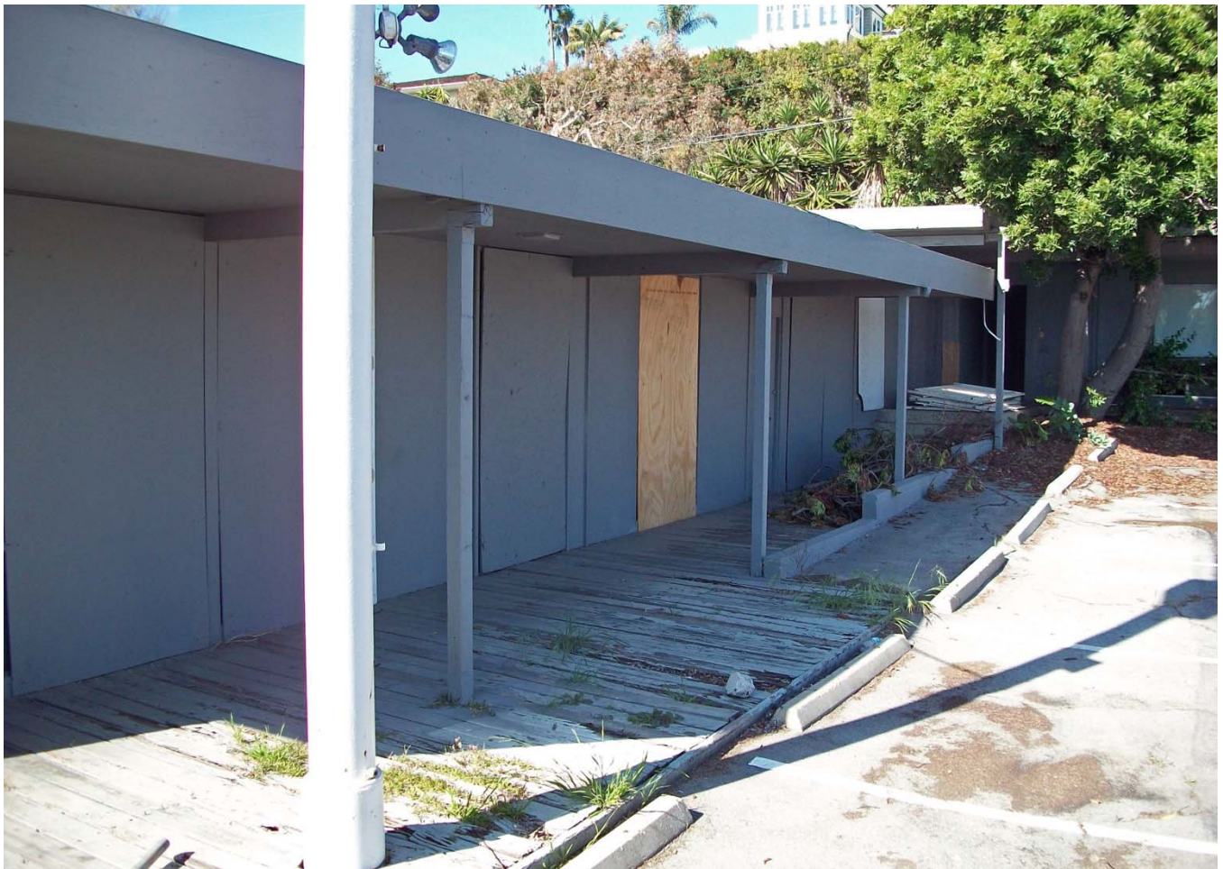
14. View of Interior Ell, West Side of Property (Northwest).
