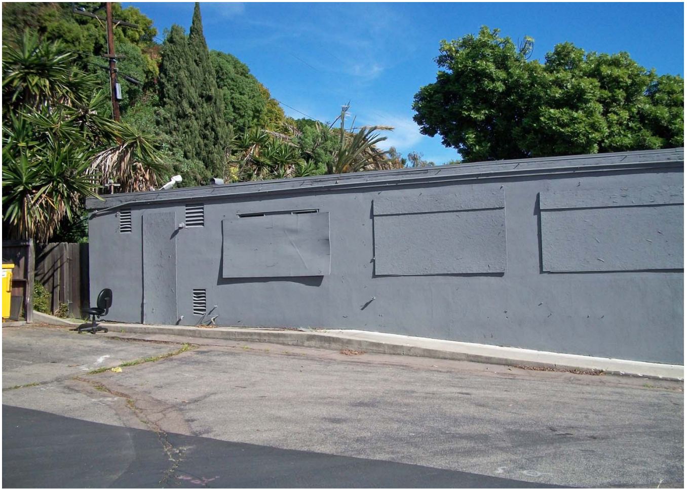
9. Detail of West Elevation in Northwest Corner of Property (East).
