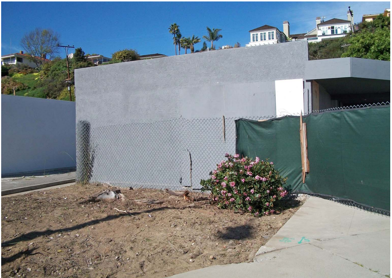
4. Flat Elevation at Southwestern Corner of Property (Northwest).
