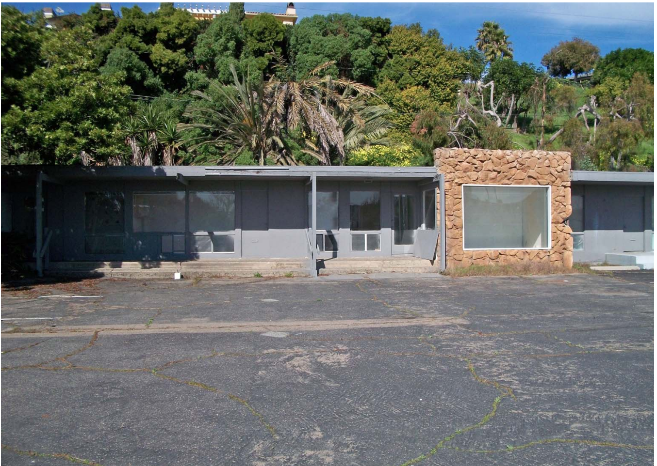
16. Overview of South Elevation, Central Portion of Property (North).
